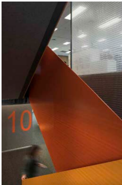
↑ ABOVE: The screen was fabricated and installed as one piece and integrates with security doors at the bottom level.
