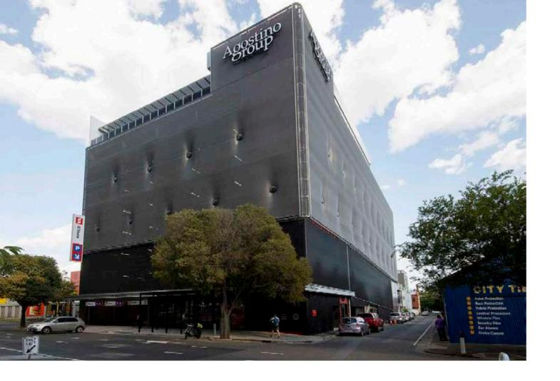
Inspired by an old leather couch the architect's unique concept called for button-like discs to be pulled back into the Kaynemaile mesh. To get the design right we prototyped the concept at scale, making sure it could be successfully realised and installed within the fast installation schedule.
