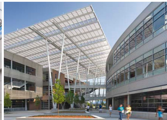
▲ Project: UNF Student Center id 24863 Location: Jacksonville, FL Architect: Rink Design Partnership
