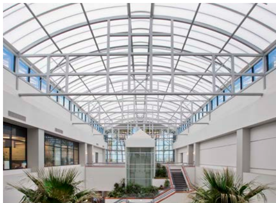
▲ Project: Hologic, Inc. id 34563 Location: San Diego, CA Architect: Smith Group Consulting
